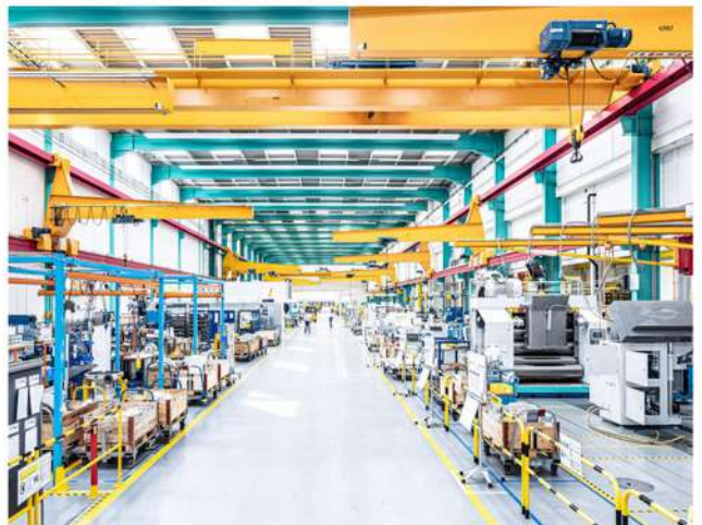
ELECTRICAL & MECHANICAL SUPPLY
